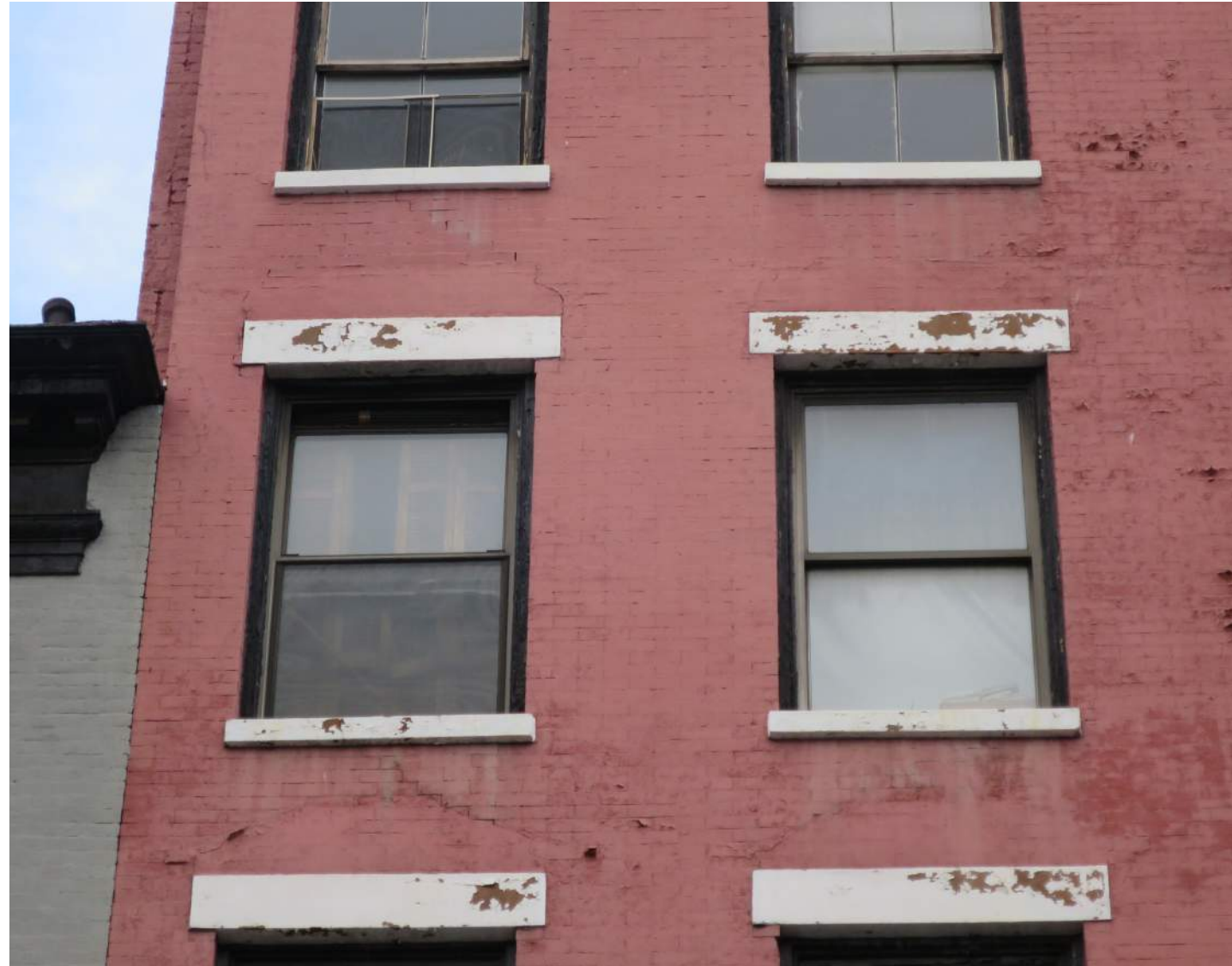
THIRD-FLOOR ALUMINUM WINDOWS
