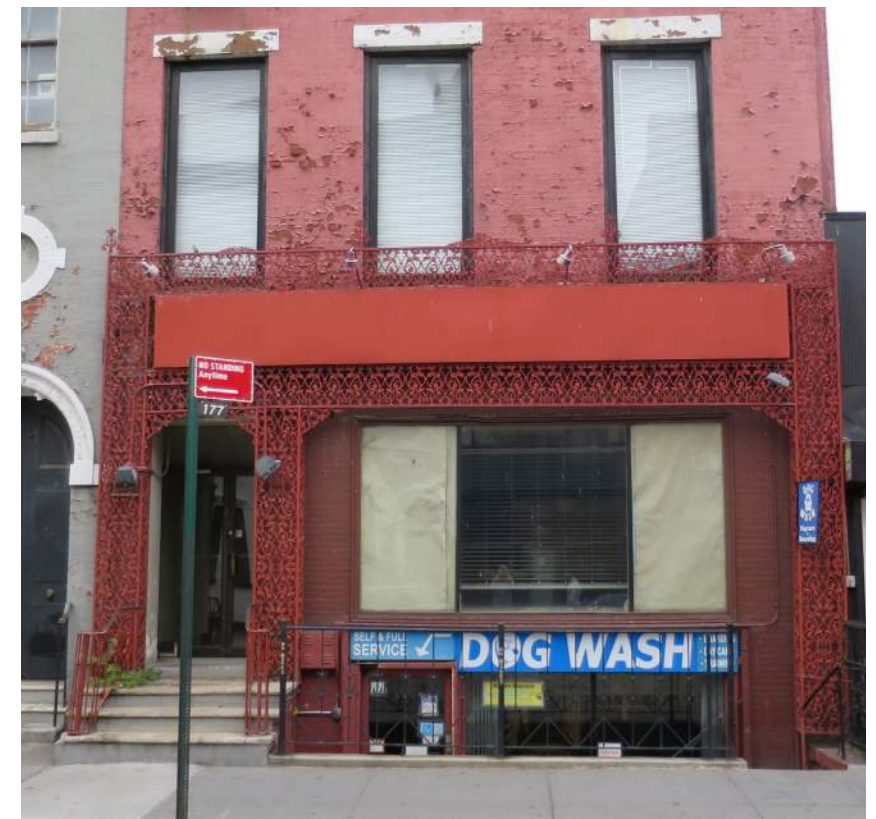
NON-HISTORIC CAST-IRON LATTICE
