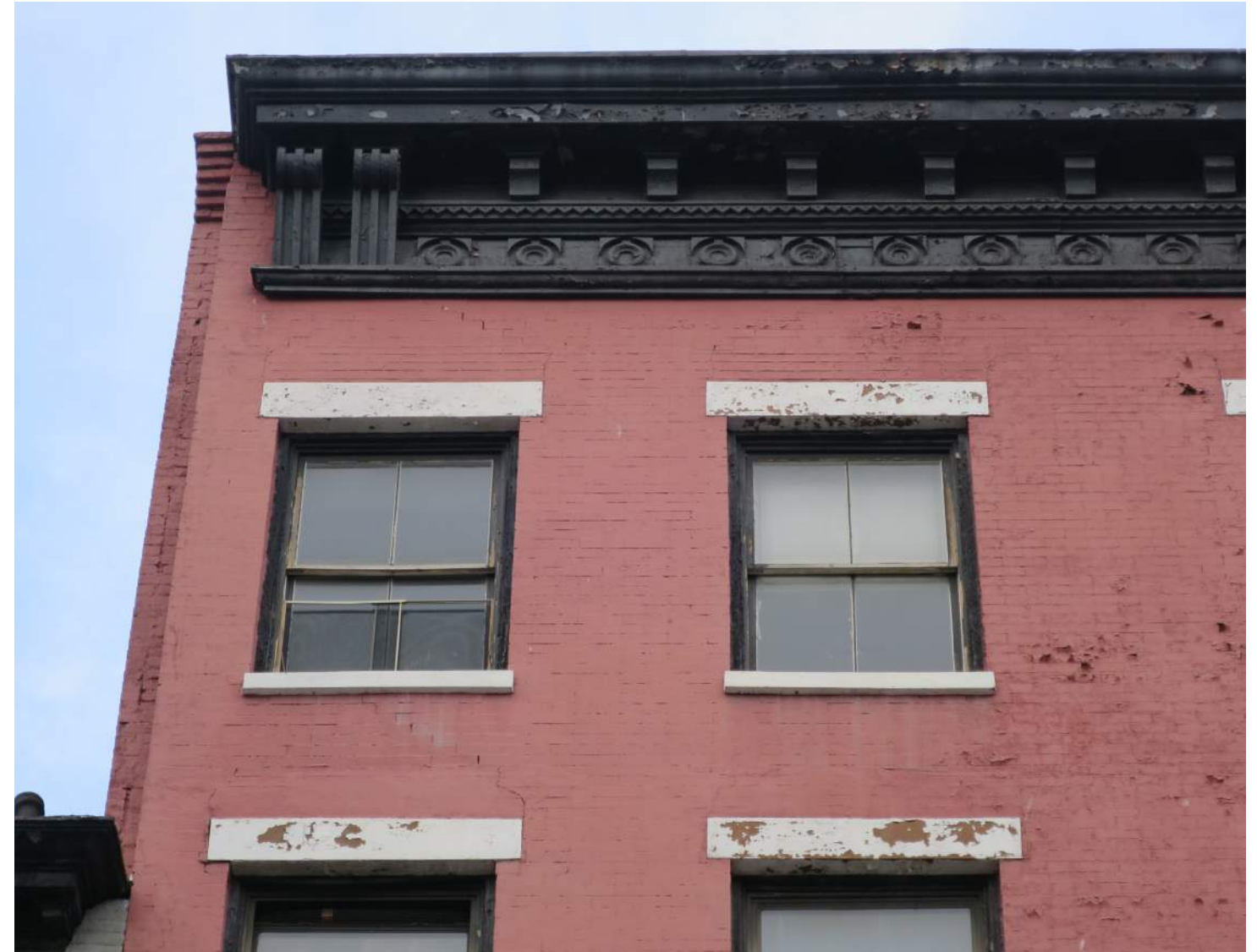
HISTORIC METAL CORNICE AND DETERIORATED WOOD WINDOWS
